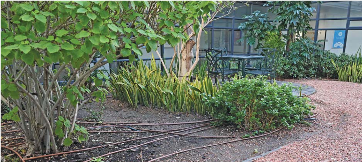
Figure 19: Drip irrigation systems support effective water management by delivering water directly to plants with minimal waste, promoting sustainable gardening practices.
